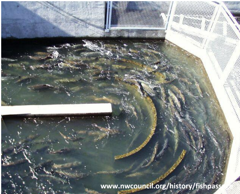
Bonneville Dam fishway Columbia River, Washington
